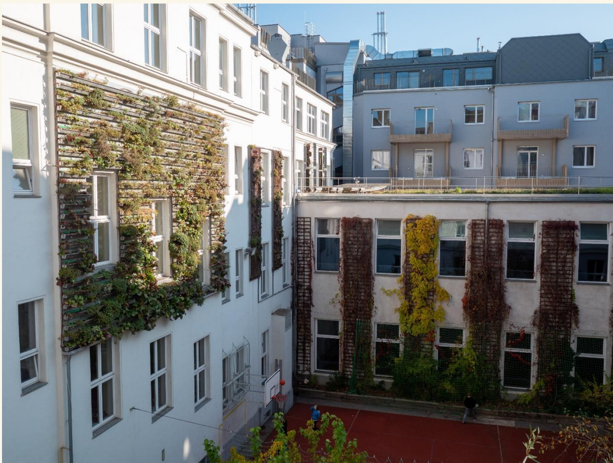
Figure 25. Outdoor green walls at GRG7 Kandlgasse. Source: © PPMI, 2024. Photographer: Gabriel Kudela.
