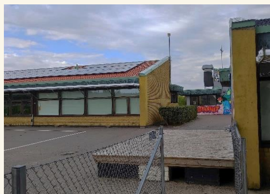
Figure 12. Solar panels on the roof at Gantofta school.
